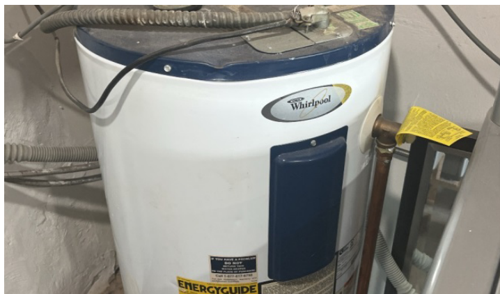
Existing Water Heater Before Wrap
