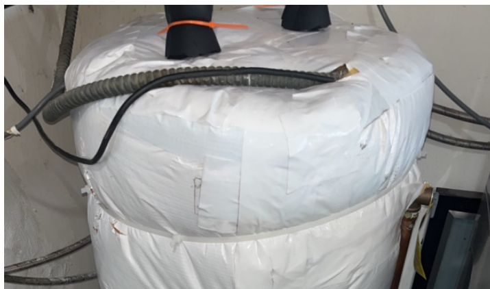
Water Heater with Wrap
