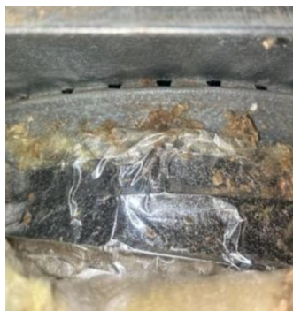
Duct Sealing Before
