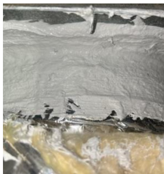
Duct Sealing After
