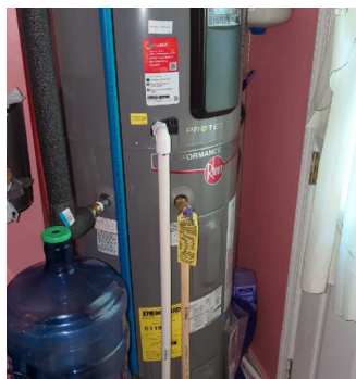
New Heat-Pump Water Heater
