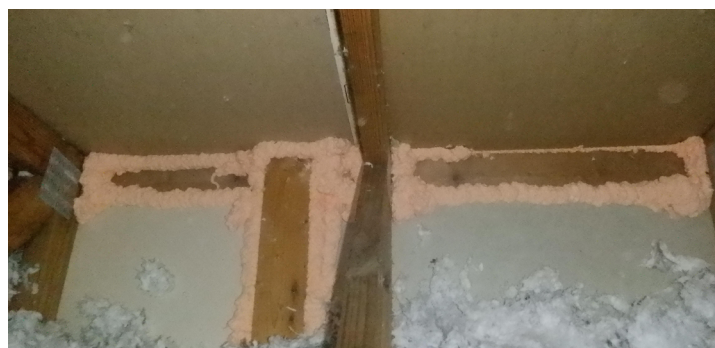
After Air Sealing
