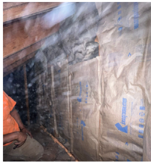
Insulation Installed
