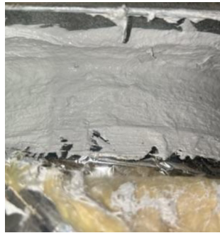
Duct Sealing After
