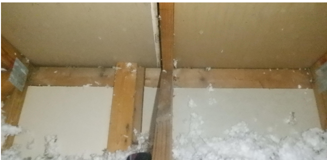
Before Air Sealing
