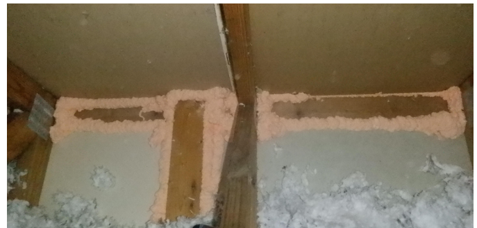
After Air Sealing
