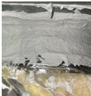
Duct Sealing After
