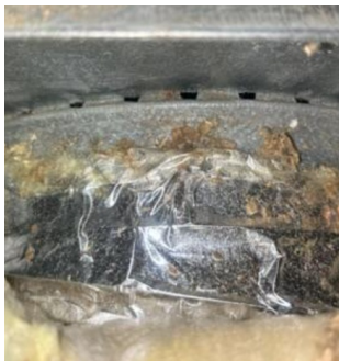
Duct Sealing Before
