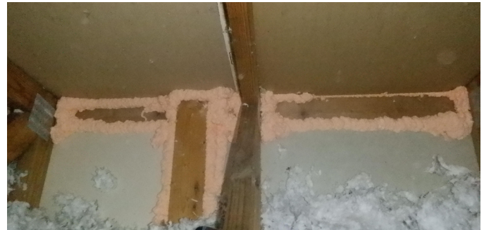
After Air Sealing
