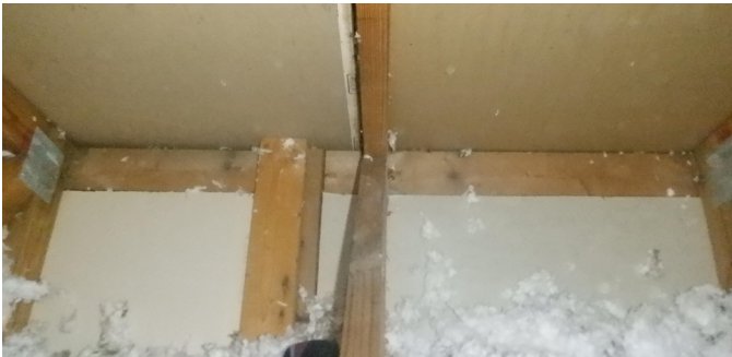
Before Air Sealing
