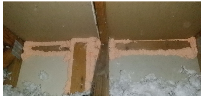
After Air Sealing
