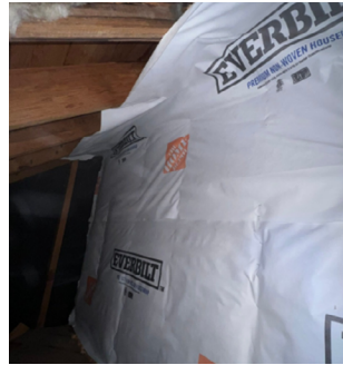
Insulation Installed
