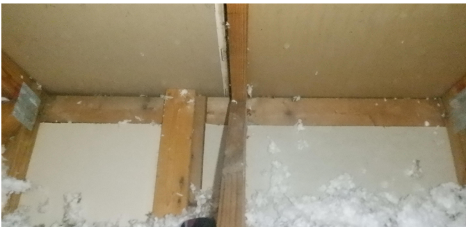
Before Air Sealing
